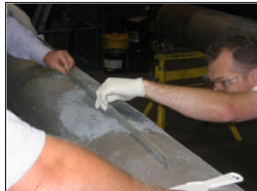
Fig. 4 – Use a straight edge to confirm evenness.
