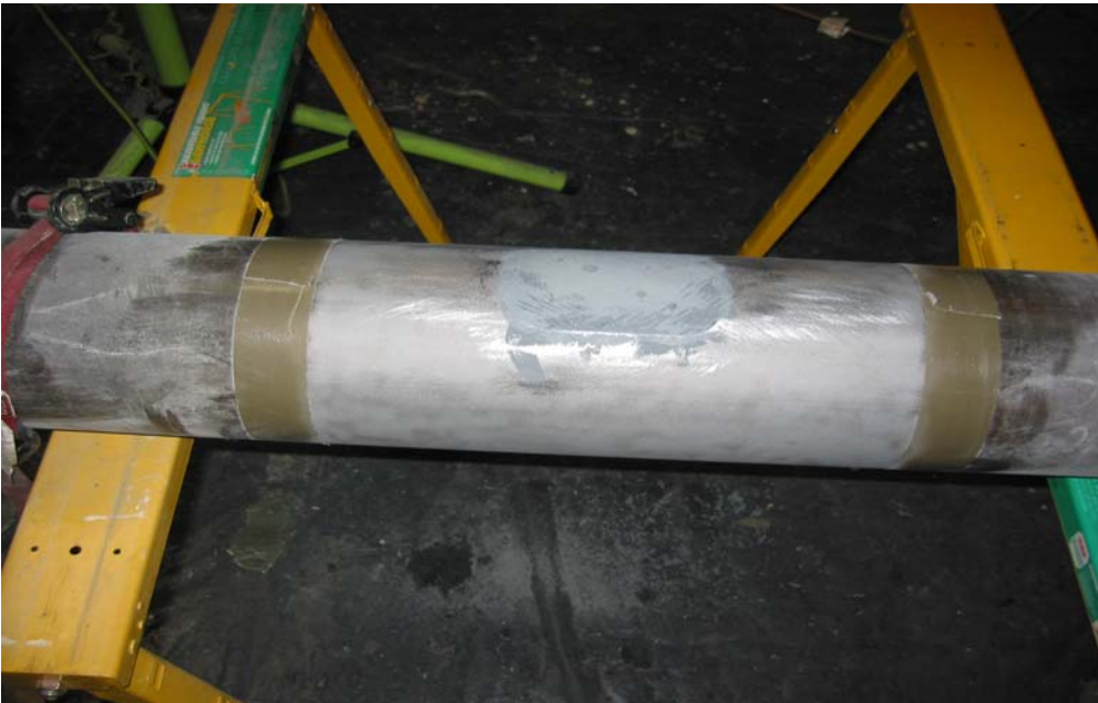
Photo 2. Pipe with load transfer material installed
