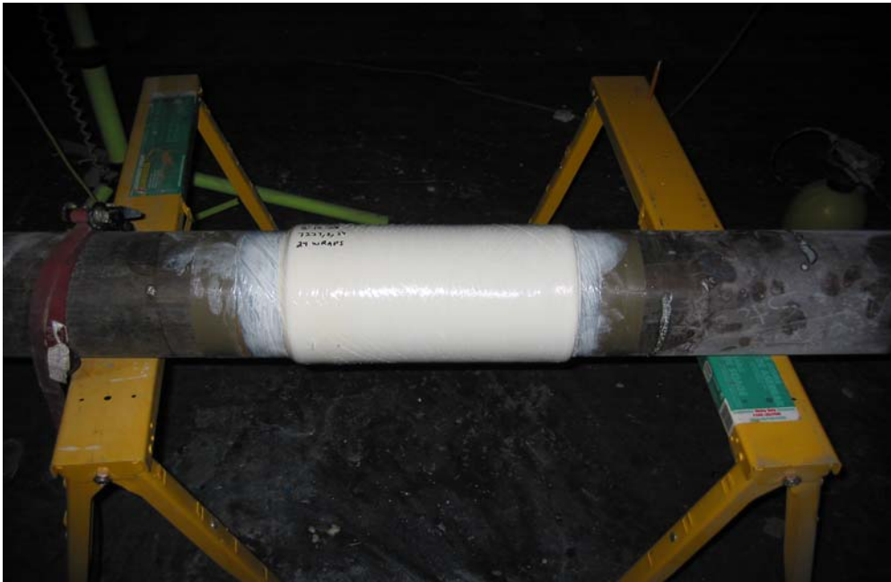
Photo 4. Pipe with wrap installed
