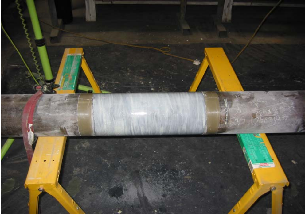
Photo 3. Pipe with adhesive
