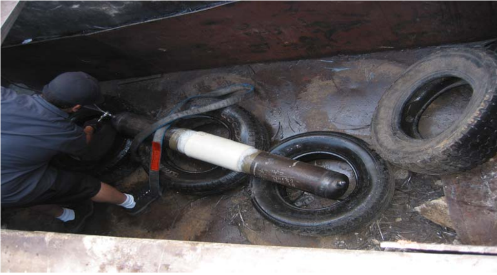
Photo 5. Wrapped pipe in test pit.
