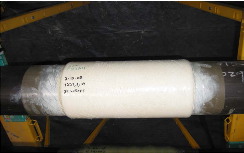
Photo 6. Pipe section after successful test.
